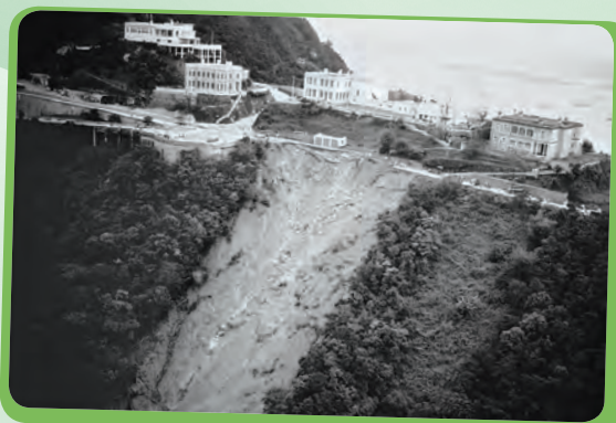
1966年山頂道山泥傾瀉 – 主要道路中斷 Peak Road Landslide in 1966 – Major road damaged
