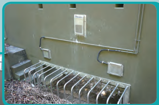
深井新村泥石壩的山泥傾瀉偵察系統 Landslide detection system installed on a rigid barrier in Sham Tseng San Tsuen
