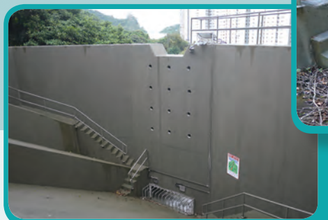
深井新村泥石壩的山泥傾瀉偵察系統 Landslide detection system installed on a rigid barrier in Sham Tseng San Tsuen
