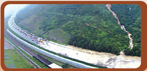
2008年北大嶼山公路天然山坡山泥傾瀉，導致通往香港國際機場的主要幹道被封閉約16小時 North Lantau Highway Natural Terrain Landslide in 2008, resulting in closure of major transport corridor to the Hong Kong International Airport for about 16 hours
