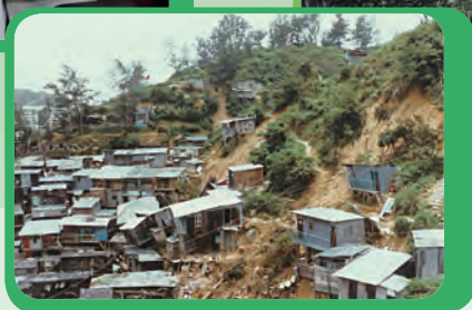
清拆山區寮屋 Clearing hillside squatters
