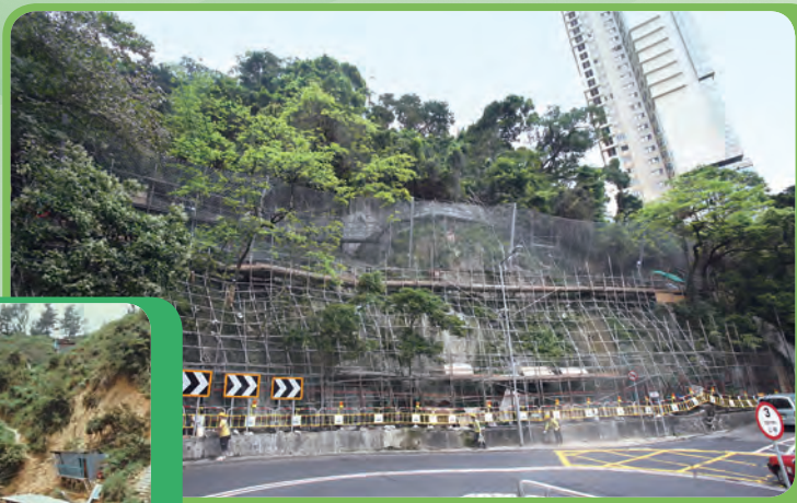
鞏固不合標準斜坡 Upgrading substandard slopes
