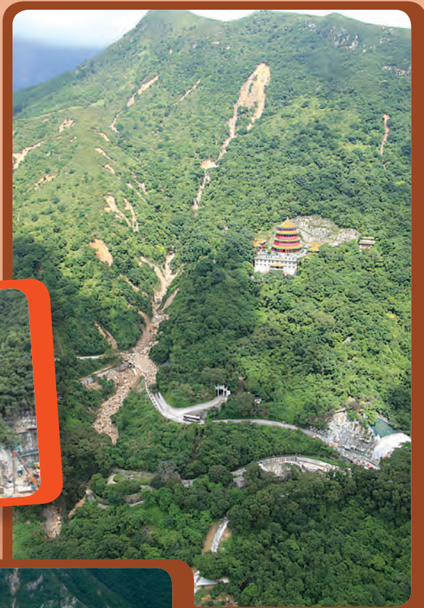
2008年羌山道天然山坡山泥傾瀉，導致通往大澳的道路被封閉14天 Keung Shan Road Natural Terrain Landslide in 2008, resulting in closure of access road to Tai O for 14 days
